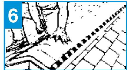
Install new ridge cap in normal manner, using 2-1/2" roofing nails, for 3/4" deck penetration or penetration through the deck, whichever is less. Nailing the ridge caps through the vent along the nailing line will secure the vent. Shingles may need to be trimmed.
