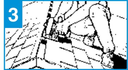
Cut along chalk lines. Remove roof sheathing. **Note:** Slot should not be cut any closer than within twelve (12) inches of gable end, hip intersecting ridge.
